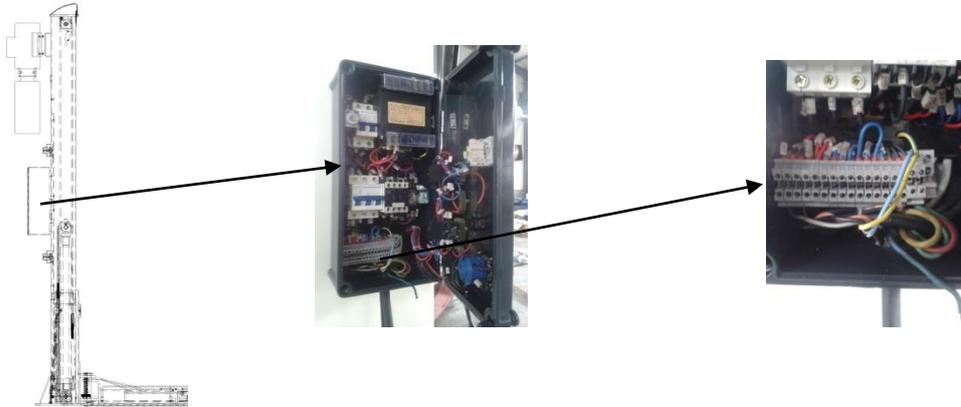
2. Connect the limit switch on the main Column. (NB. Note the misalignment of the limited switch within the column!)
